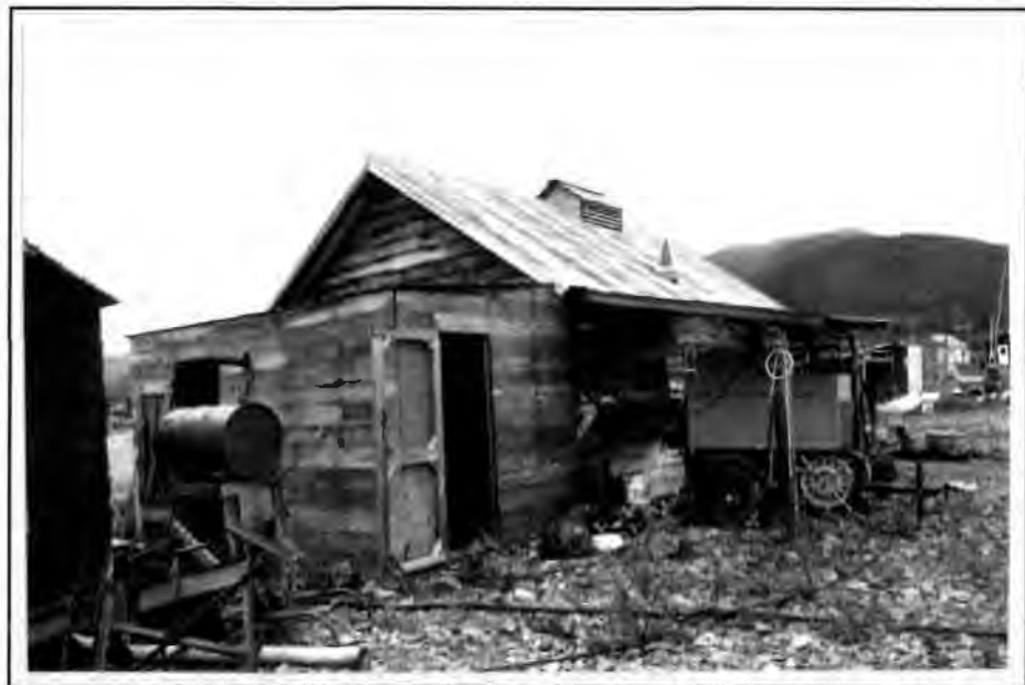
Figure 148. The Golden Horn Powerhouse, 1993. The view is looking northwest.
